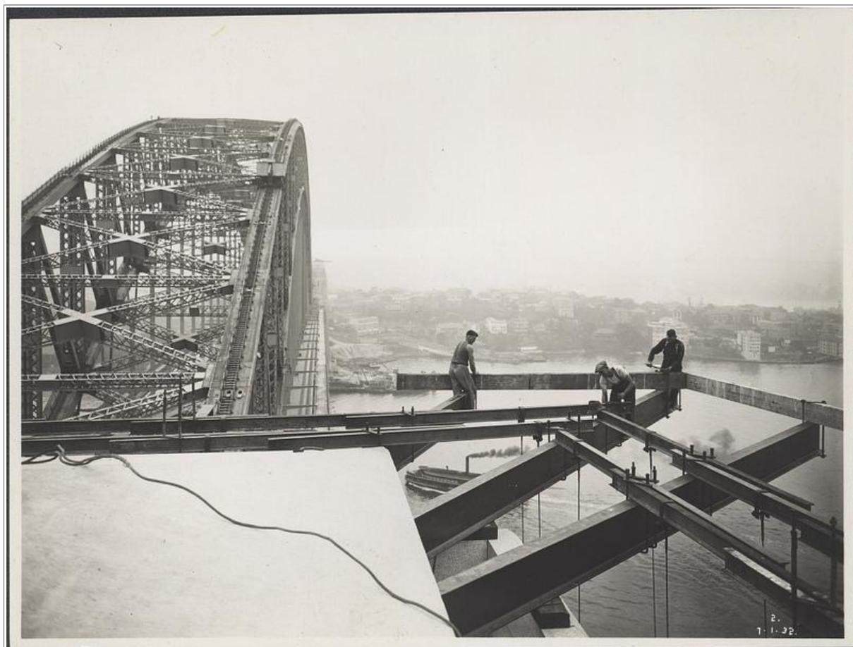
Workmen attaching the supports to a pylon of the Sydney Harbour Bridge.
