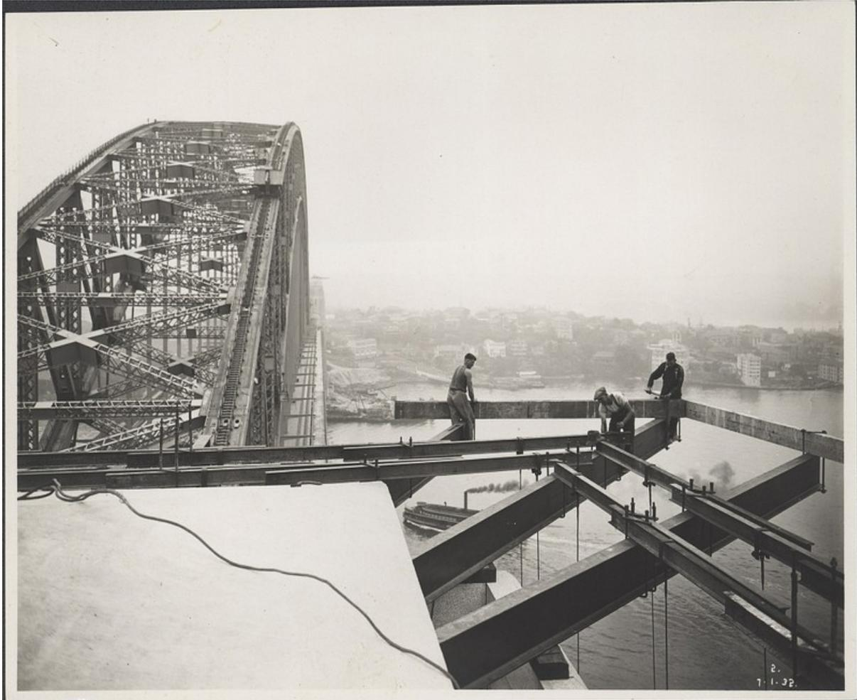
*Workmen attaching the supports to a pylon of the Sydney Harbour Bridge.*
